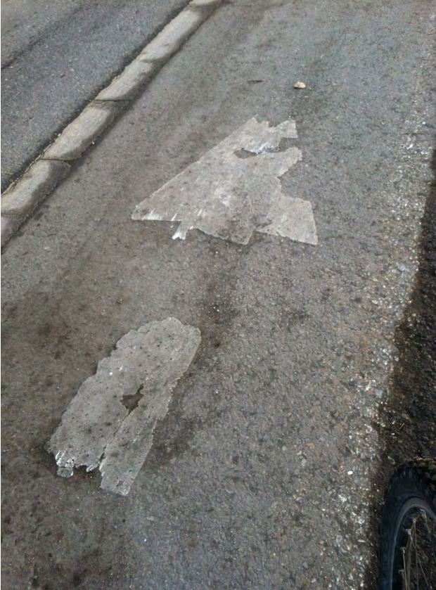
Thermoplastic marking scraped off by plow blade in Bozeman, MT
