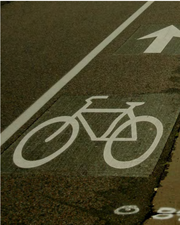
Recessed thermoplastic markings in Minneapolis, MN
